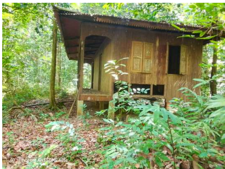
Abandoned chalets within Taman Negara NP close to Sungai Sepia that could be refurbished with local management
